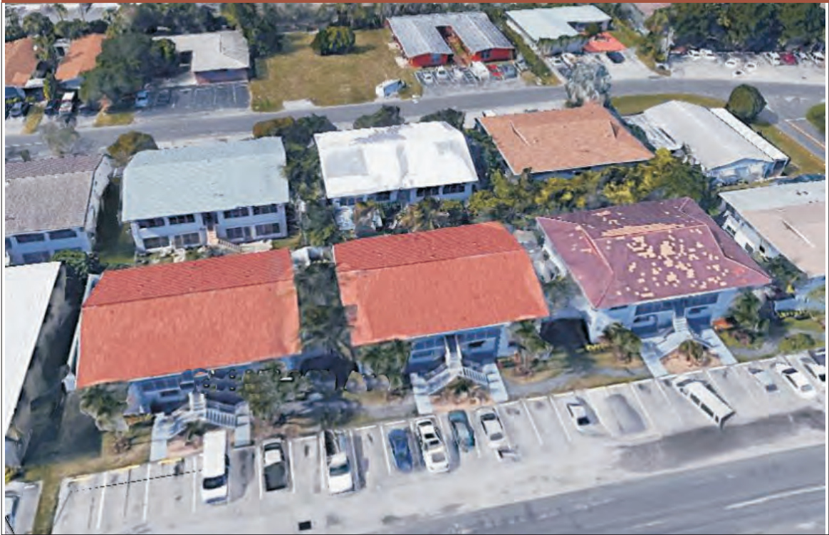
Figure 11: Cluster of Four Clustered Recovery Communities in Nearby Pompano Beach
