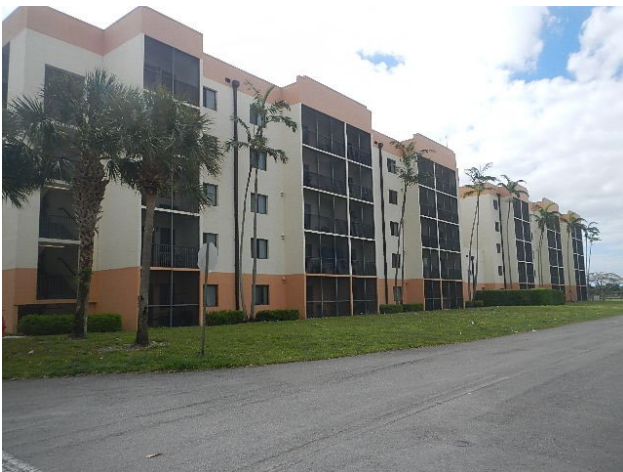
View SE at NWC of Tower II
