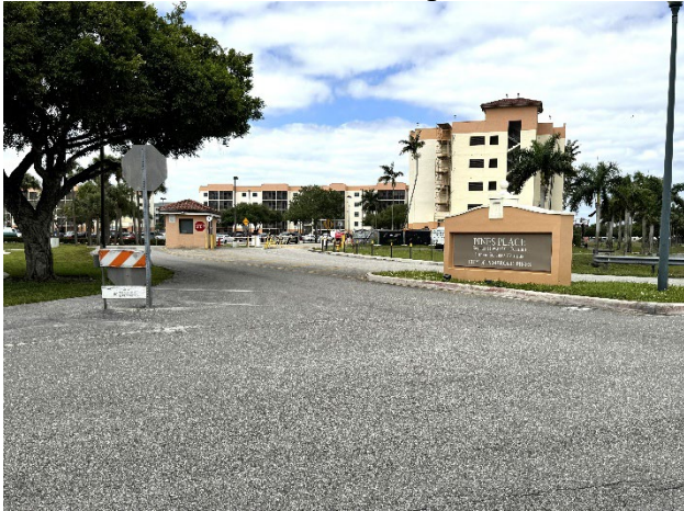
View NW at Entrance to Complex
