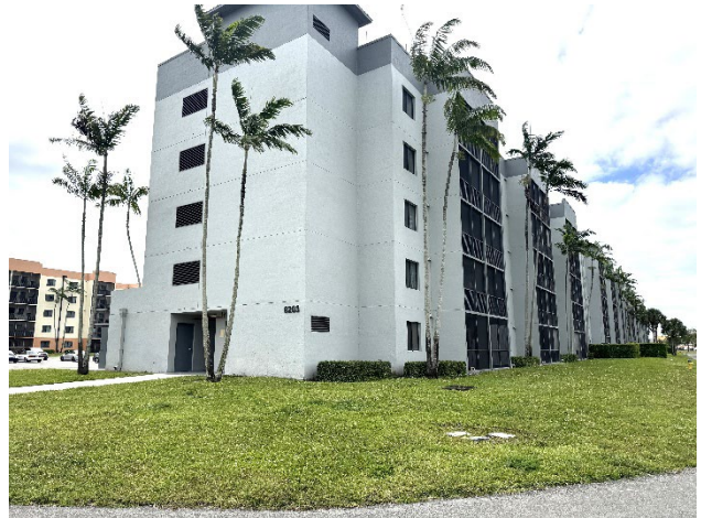
View NW of SEC of Tower III
