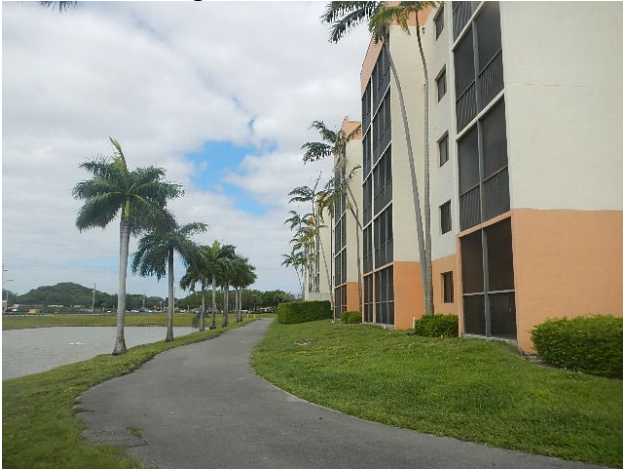
View S of completed renovations to Tower II
