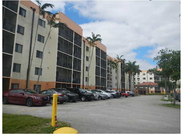
View W of NEC of Tower II-renovated portion
