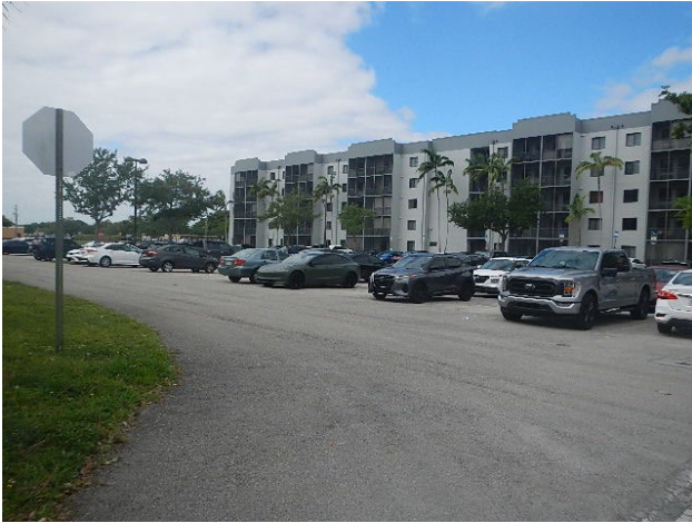
View SW at NEC of Tower III
