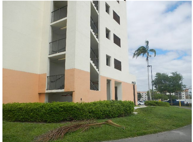
View SW of Tower II-Northerly Elevation
