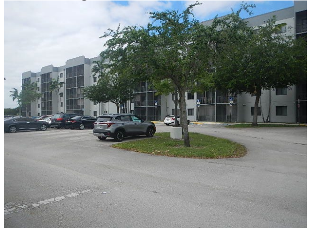
View S along W side of Tower III
