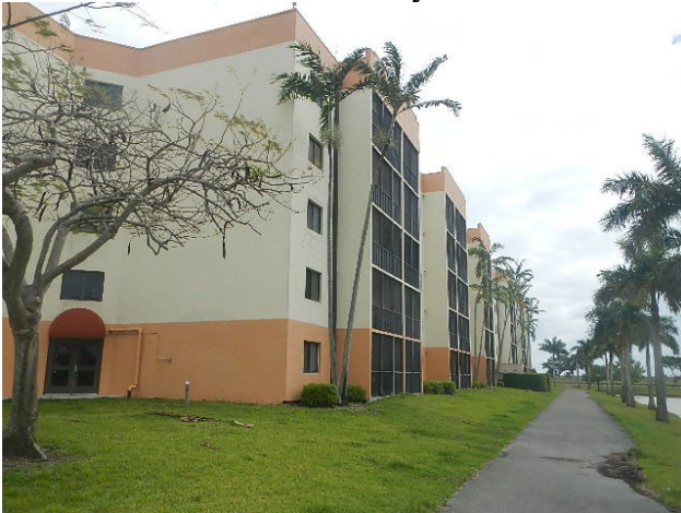
View N of Tower II-Southerly Elevation
