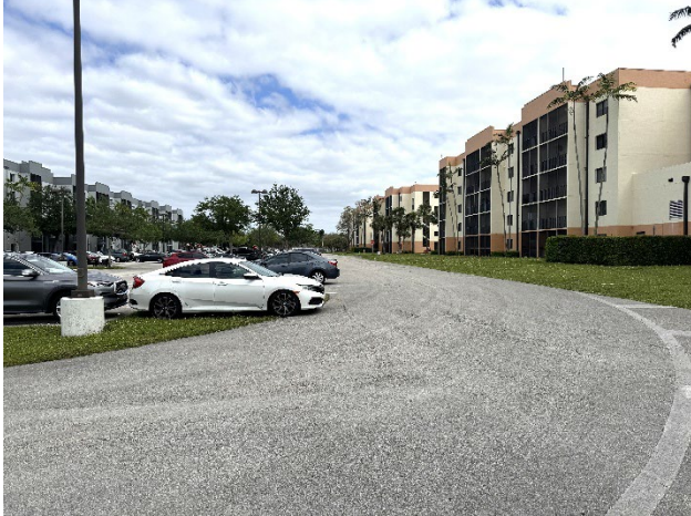
View SW along Palm Dr. showing Tower I
