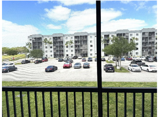
View SE at NWC of Tower III
