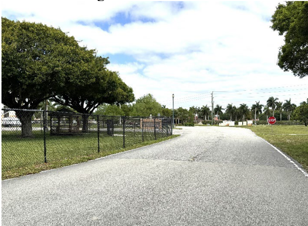
View NW along Palm Dr. near entrance
