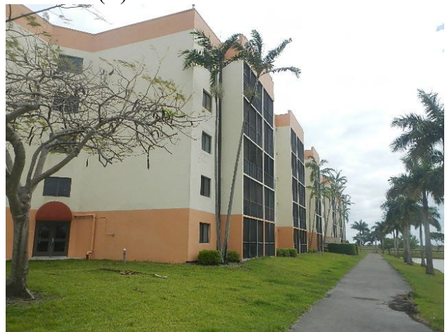
View S across parking showing Tower II (L) & Tower III (R)
