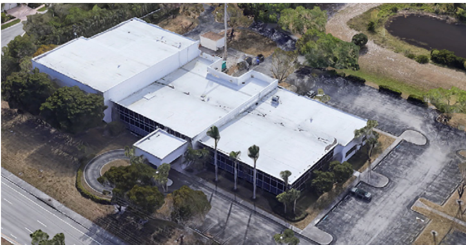
WXEL-TV/PBS Roof Replacement, Boynton Beach
