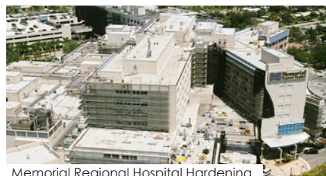
Memorial Regional Hospital Hardening
