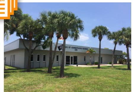
Lantana Motorists Renovation
