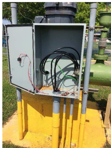
Figure 2b: Well 9 Junction Box with E-Stop
