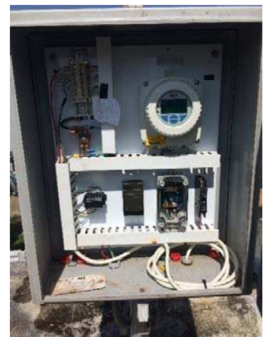
Figure 1c: Well 6 Flow Meter Enclosure
