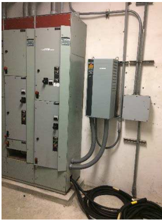
Figure 5i: Control Building – VFDs Well 10 and Generator Cables
