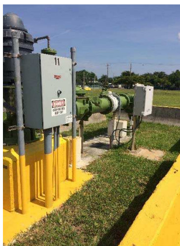
Figure 4b: Well 11 Junction Box with On/Off Switch
