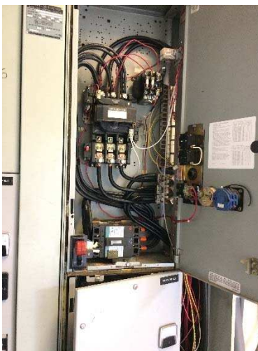
Figure 5k: Control Building – Well 9 MCC Cubicle
