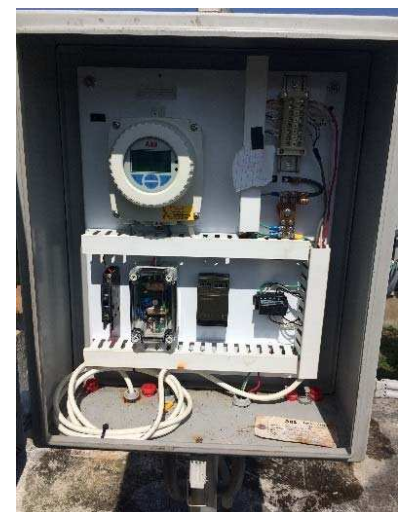
Figure 3c: Well 10 Flow Meter Enclosure
