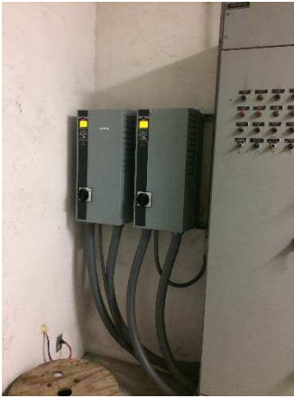
Figure 5g: Control Building – VFDs Wells 9 & 11
