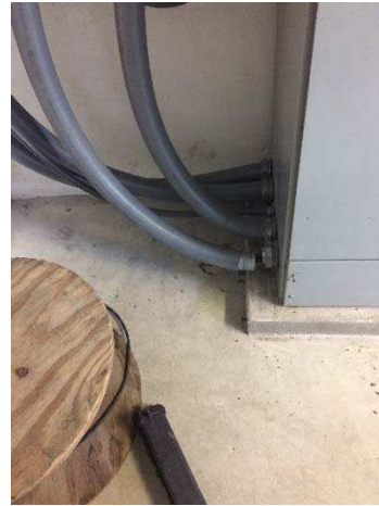
Figure 5h: Control Building – Broken Conduit for Well 11 VFD
