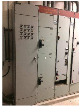
Figure 5j: Control Building – MCC
