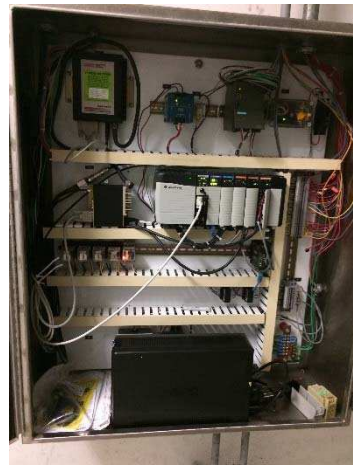
Figure 5f: Control Building - RTU
