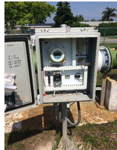
Figure 2c: Well 9 Flow Meter Enclosure
