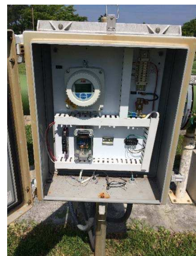
Figure 4c: Well 11 Flow Meter Enclosure
