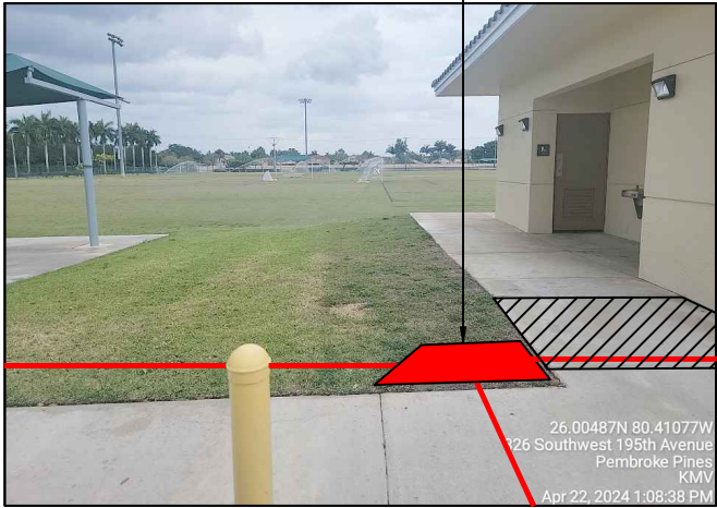
STA 18+60 INSTALL PEMPROKE PINES HANDHOLE
