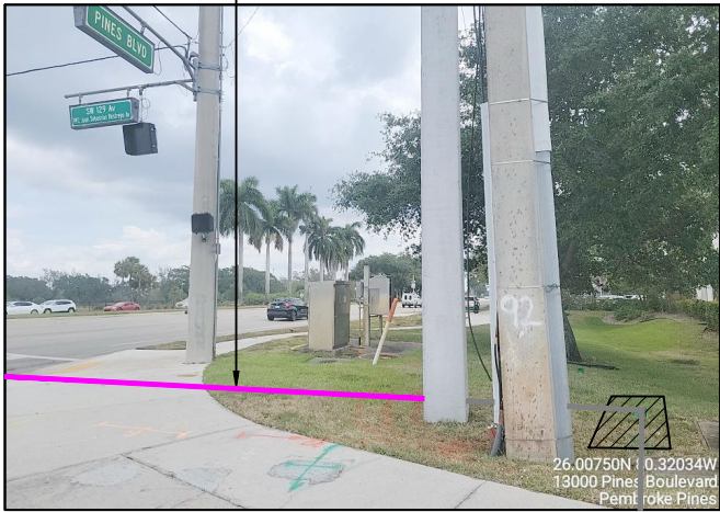
STA 2+35 DIRECTIONAL BORE
