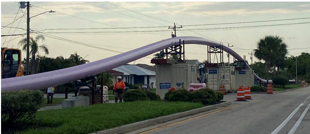
Figure 5. Aerial Pipe Support to Allow Traffic to Pass Beneath during Pullback
