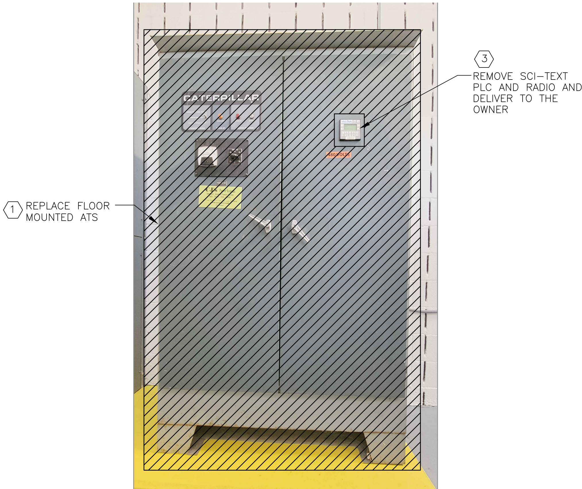
PHOTO 1: ATS DEMOLITION – FRONT VIEW
