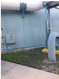
F. REROUTE AIR HEADER TO AVOID BLOCKING MANWAY AND CONNECT TO EXIST. AIR HEADER
