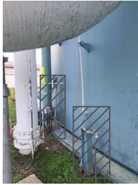
B. ABANDONED AIR HEADER PRESSURE GAUGE AND EXIST. HOSE BIBB
