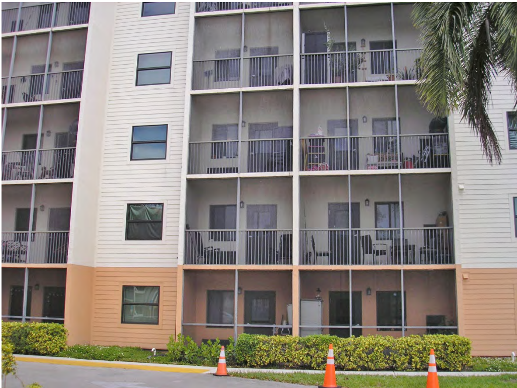
P 24 8210 Repaired Wall Sections
