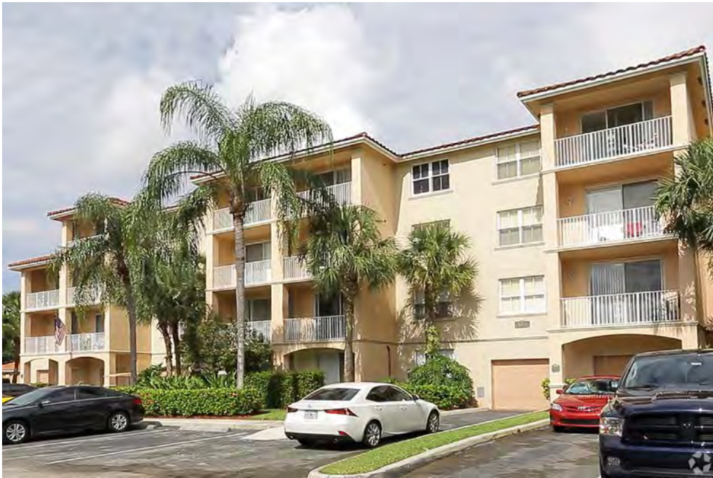
Rental 3 Falls of Pembroke Apartments
