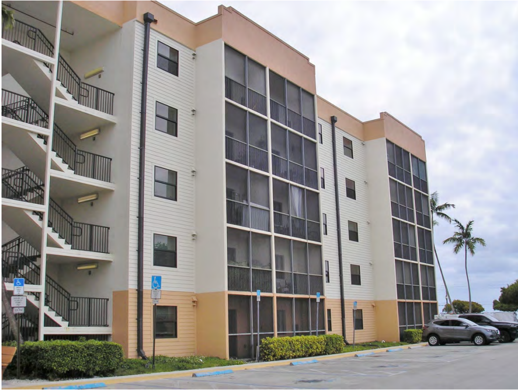
P25, 8210 East Section of South Wall
