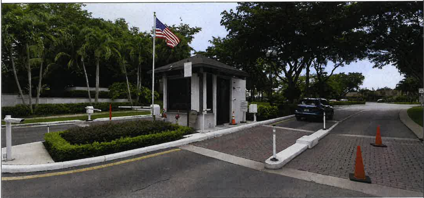
Gatehouse – South & East
