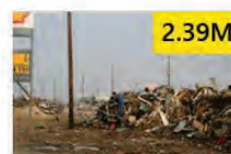
2.39M Harris County, TX Hurricane Ike, '08
