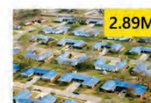
2.89M Gulfport, MS Hurricane Katrina, '05
