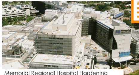
Memorial Regional Hospital Hardening
