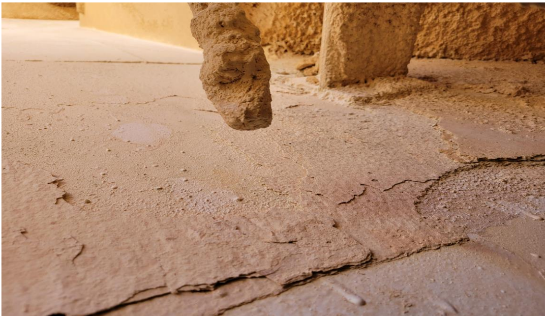
Bottom Flushing System Nozzle - Clogged
