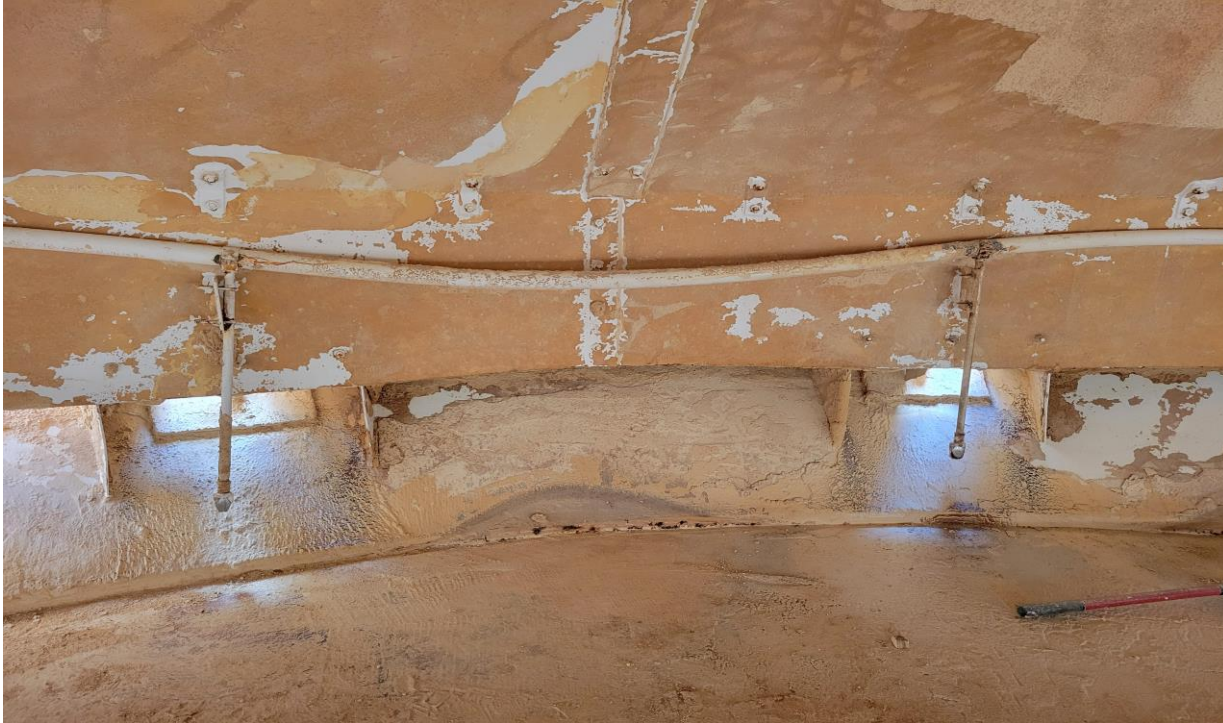
Bottom Flushing System Nozzle - Clogged
