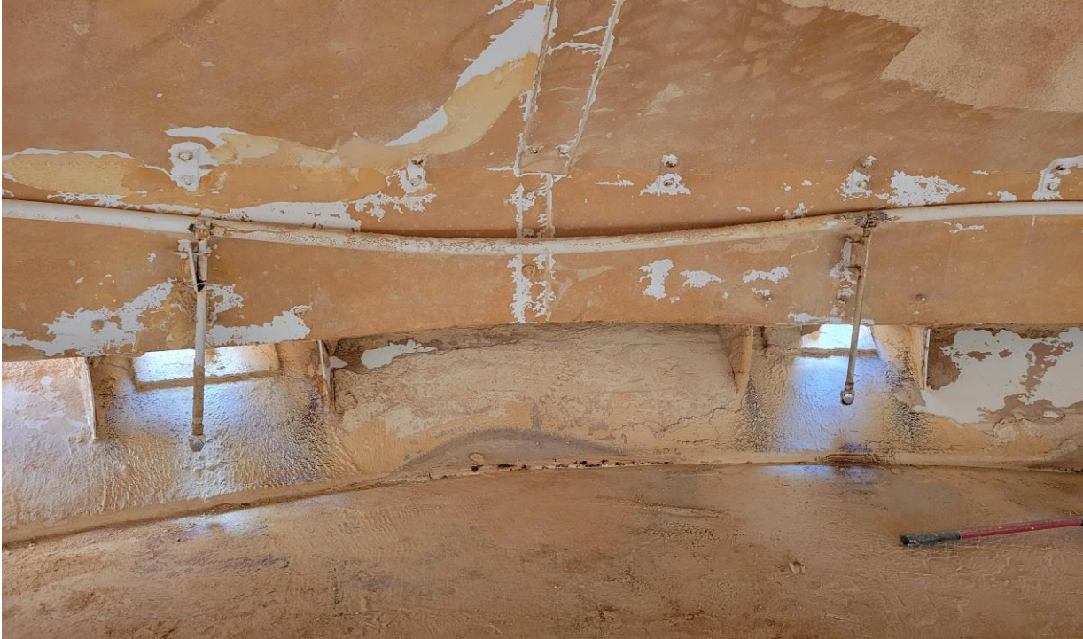
Bottom Flushing System Nozzle - Clogged
