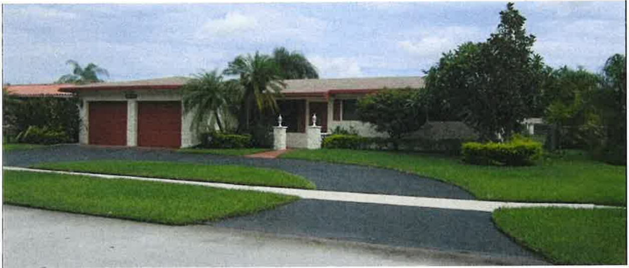
Before and After: 11911 NW 22 Street
