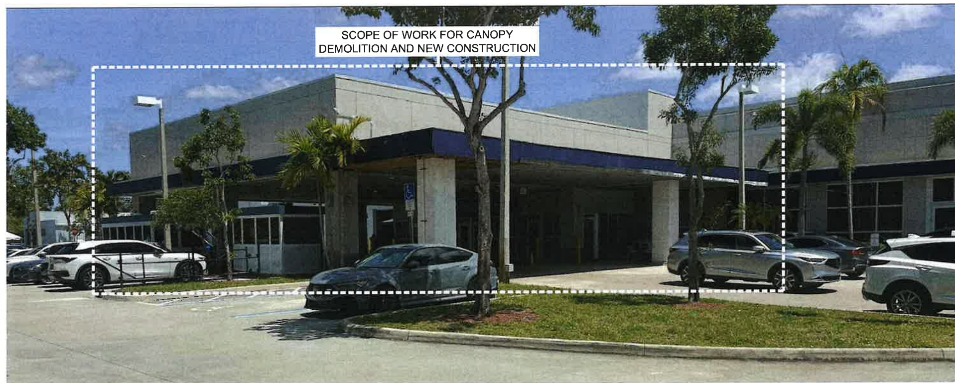
1 PHOTOGRAPH OF EXISTING WEST ELEVATION
