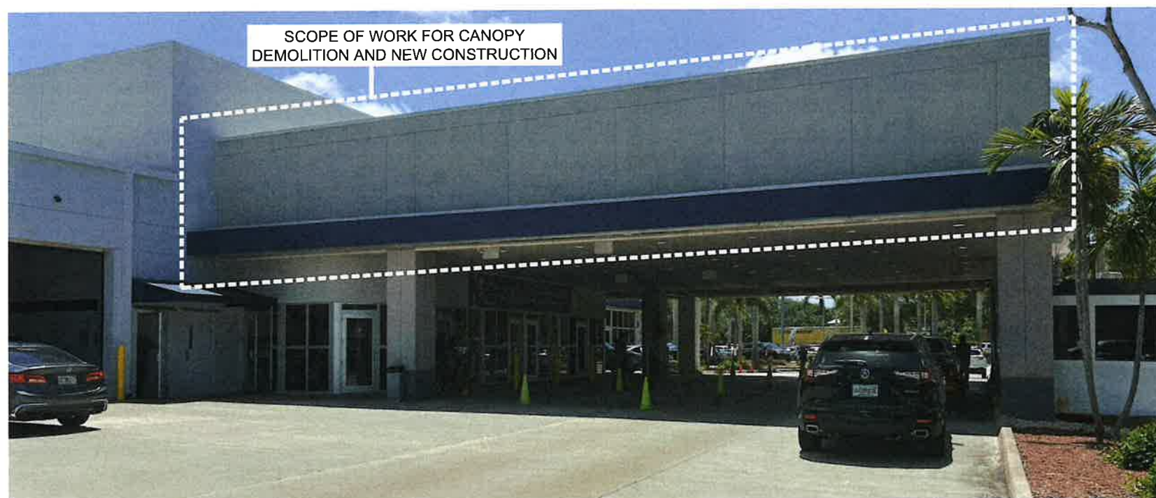
1 PHOTOGRAPH OF EXISTING NORTH ELEVATION
