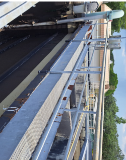
E. HANDRAIL, KICKPLATE AND WALKWAY
