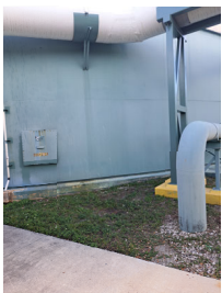
F. REROUTE AIR HEADER TO AVOID BLOCKING MANWAY AND CONNECT TO EXIST. AIR HEADER
