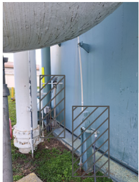
B. ABANDONED AIR HEADER PRESSURE GAUGE AND EXIST. HOSE BIBB
