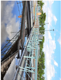
C. CLARIFIER BRIDGE AND FROTH SPRAY STEM
