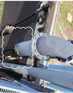
F. PIPE MOUNTING BRACKET REPAIR
