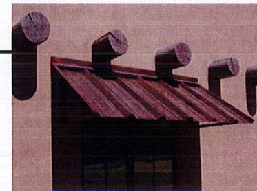
RUST FINISH AWNING
