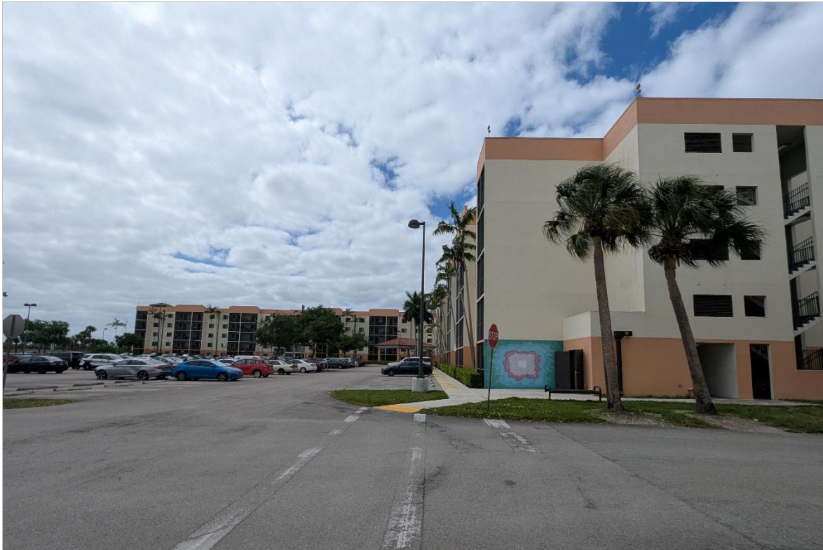
Side and front of Building 8103 (I)
