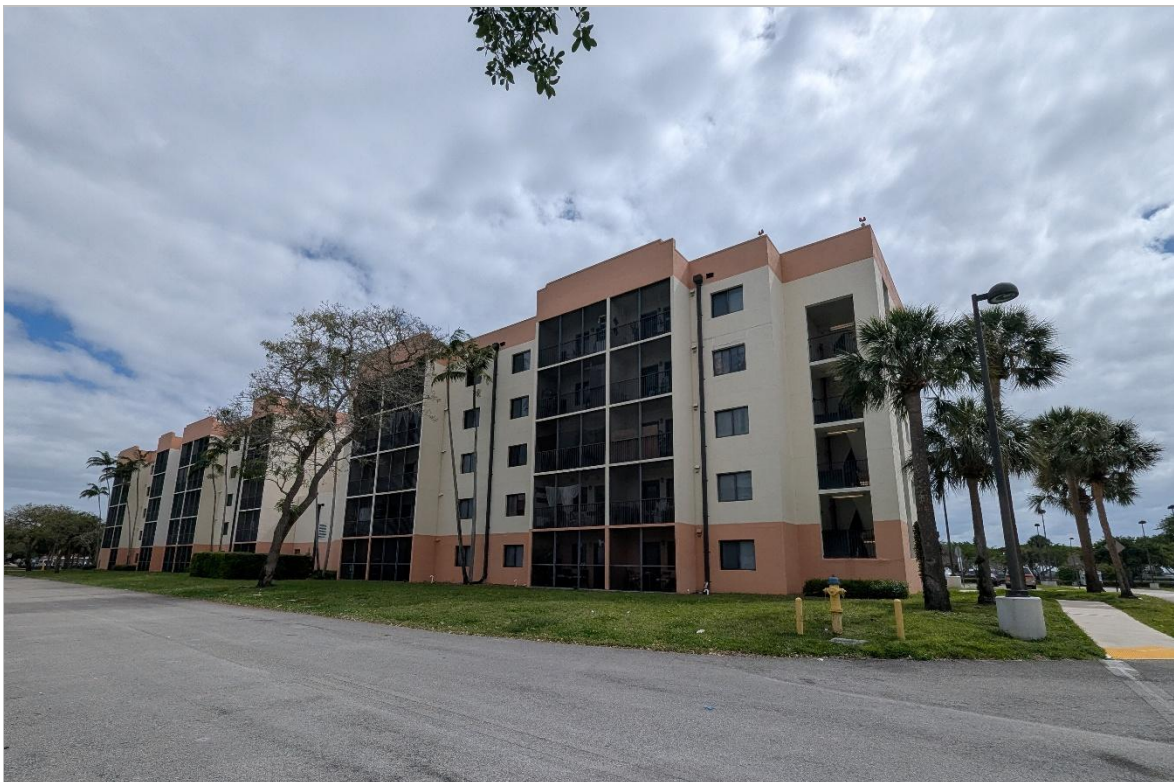
Rear of Building 8210 (II)
