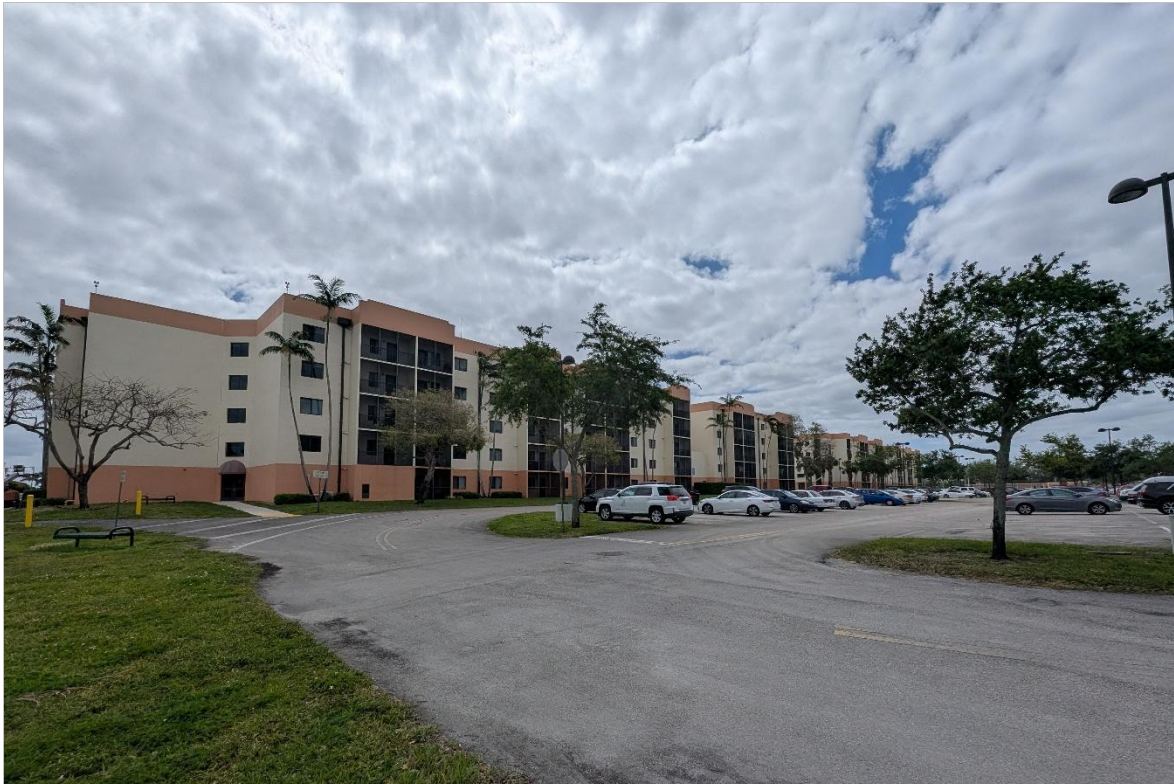
Rear of Building 8210 (II)
