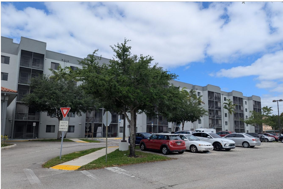
Front of Building 8203 (III)
