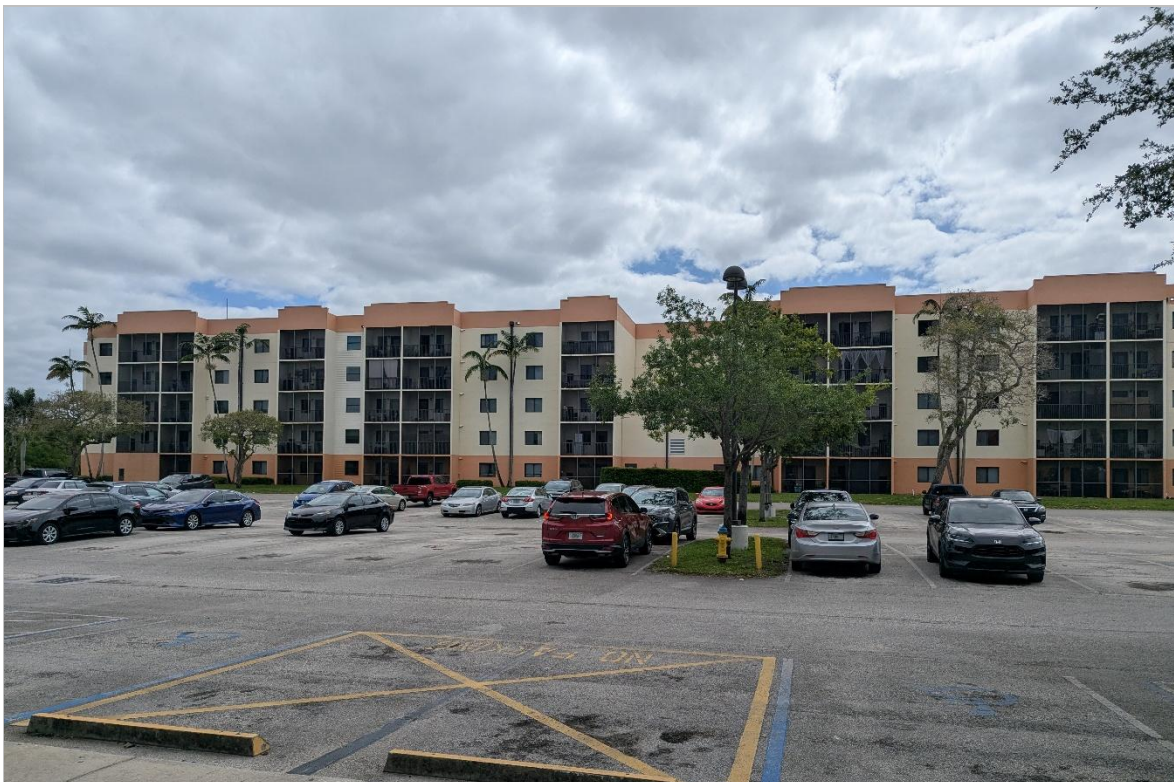
Front of Building 8103 (I)
