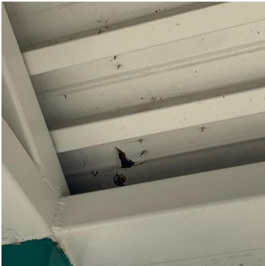
Rust/Corrosion
