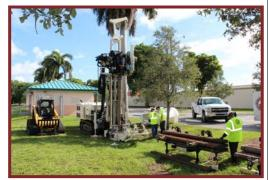
Challenges encountered Project specifications required discriminate interval water sampling of the boring to determine the conductivity and water quality to design screen interval of the well. To accomplish this GFA used an inflatable packer system designed specifically for the sonic tooling to seal off the water column and pull water samples from specific depth intervals as required by the project geologist.
