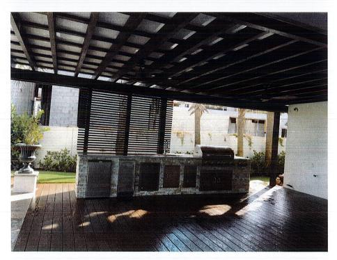
Pergola ceiling view – shows 3 inch, insulated, aluminum roof from the below, ceiling view.
