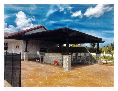
Roof is made of 3 inch, insulated, aluminum and will be in Bronze (Espresso) color to match the body of the Pergola and the roof on the home. (above is a picture of the insulated roof; it's the top layer of the Pergola.) Also, Pergola will be made of pressure treated timber and meet all code specifications.
