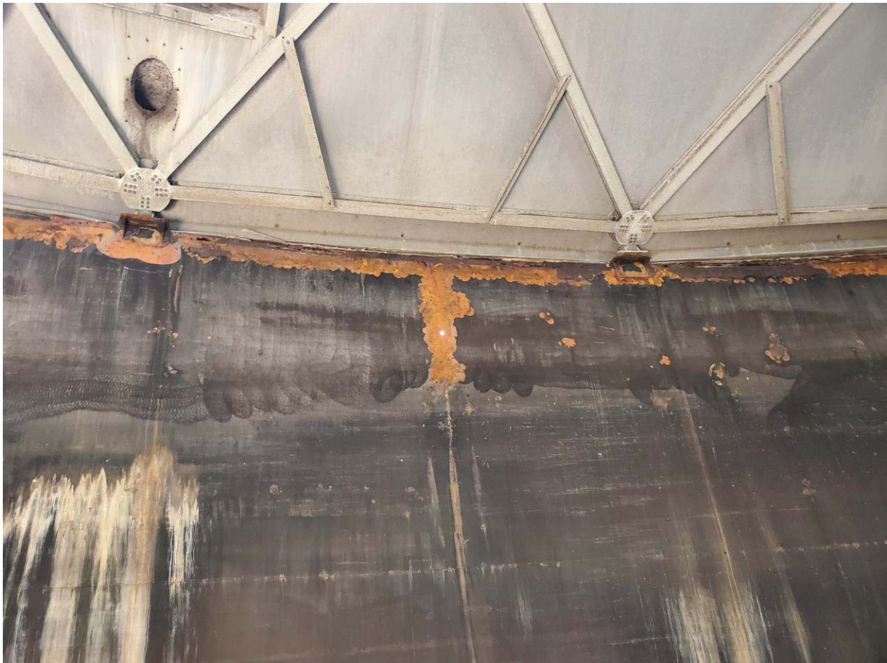
Figure 1: Visual of corrosion on upper wall sections, with noticeable hole
