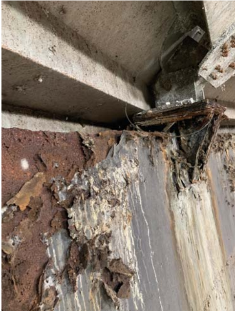
WWTP Rehabilitation East Surge Tank Corrosion Issues December 17, 2019 at 10:53:37 AM
