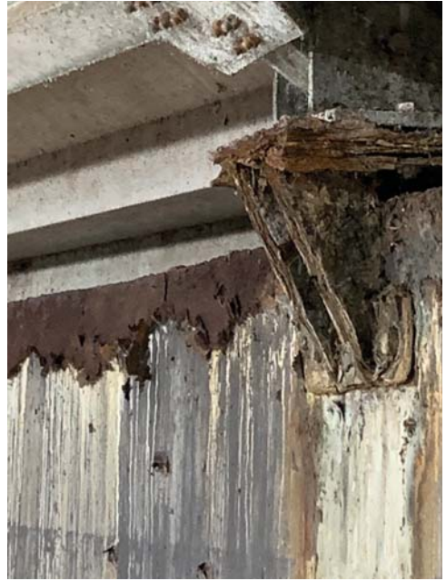
WWTP Rehabilitation East Surge Tank Corrosion Issues December 17, 2019 at 10:53:18 AM
