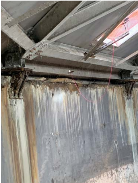
WWTP Rehabilitation East Surge Tank Corrosion Issues December 17, 2019 at 10:53:08 AM
