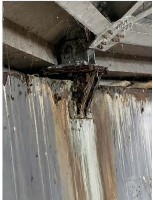
WWTP Rehabilitation East Surge Tank Corrosion Issues December 17, 2019 at 10:53:03 AM
