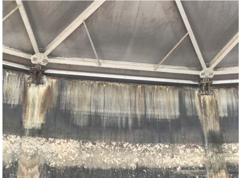
WWTP Rehabilitation East Surge Tank Corrosion Issues December 18, 2019 at 11:50:10 AM
