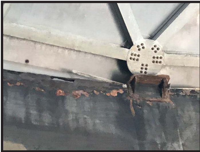
Figure 3: Dome Beam Seat Connection
