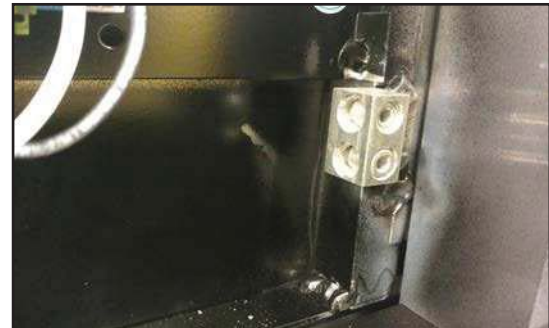
Figure 2 • Ground lug inside sign cabinet.
