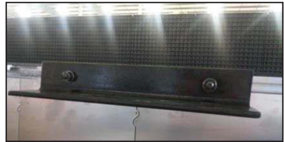
Figure 2 • Example of 18" Stringer with 1/2" bolts
