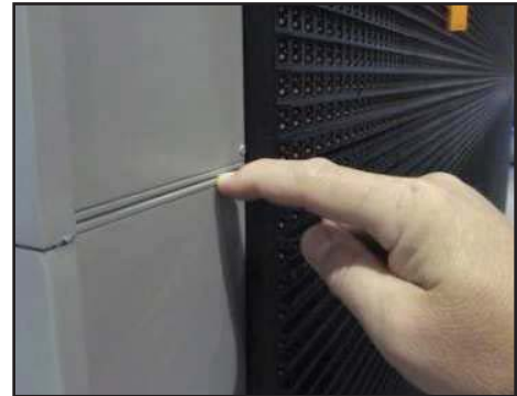
Figure 1 • Gap between cabinets.
