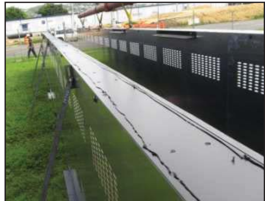
Figure 2 • Beads of silicone.
