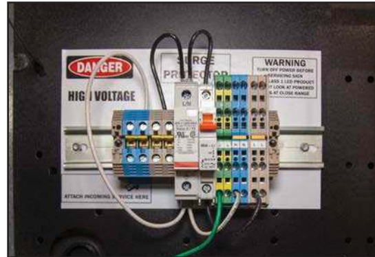
Figure 1 • 120V terminal block.
