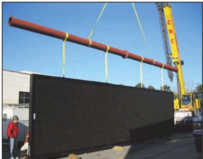
Figure 3 • Properly attached spreader bar.
