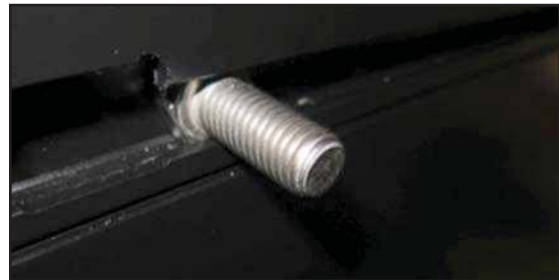
Figure 1 • Slim cabinet mounting bolt inserted in track.
