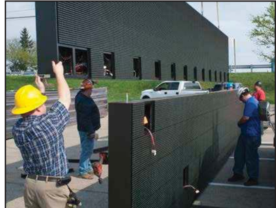
Figure 1 • Top section being placed onto lower section.
