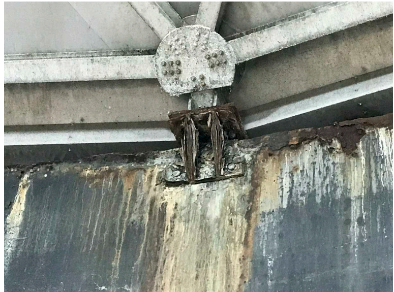
WWTP Rehabilitation East Surge Tank Corrosion Issues December 18, 2019 at 11:48:24 AM
