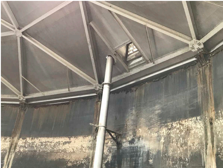
WWTP Rehabilitation East Surge Tank Corrosion Issues December 18, 2019 at 11:48:34 AM
