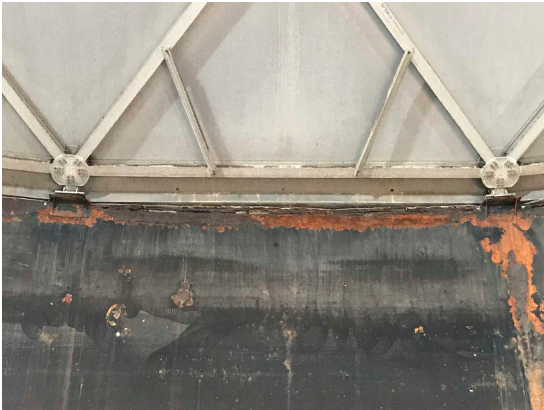
WWTP Rehabilitation West Surge Tank Corrosion Issues September 19, 2019 at 9:03:06 AM
