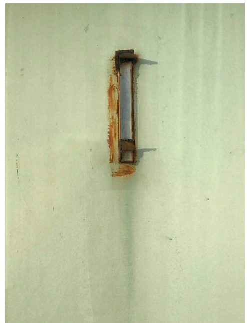
WWTP Rehabilitation West Surge Tank Corrosion Issues October 7, 2019 at 8:07:41 AM
