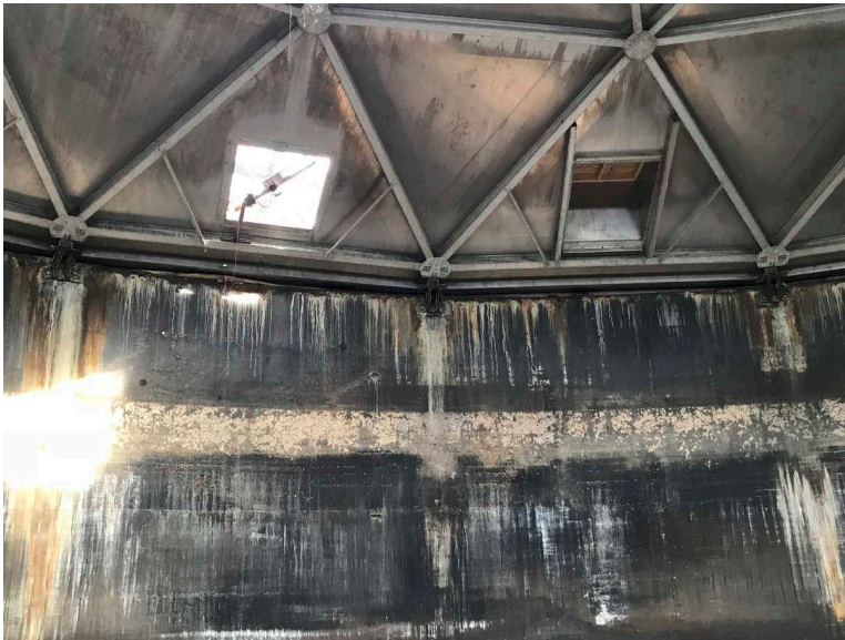
WWTP Rehabilitation East Surge Tank Corrosion Issues December 18, 2019 at 11:49:58 AM
