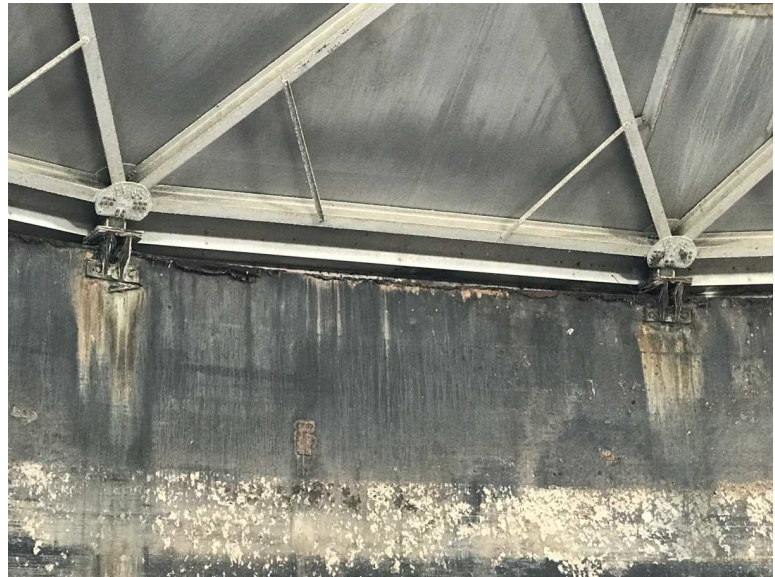
WWTP Rehabilitation East Surge Tank Corrosion Issues December 18, 2019 at 11:50:25 AM
