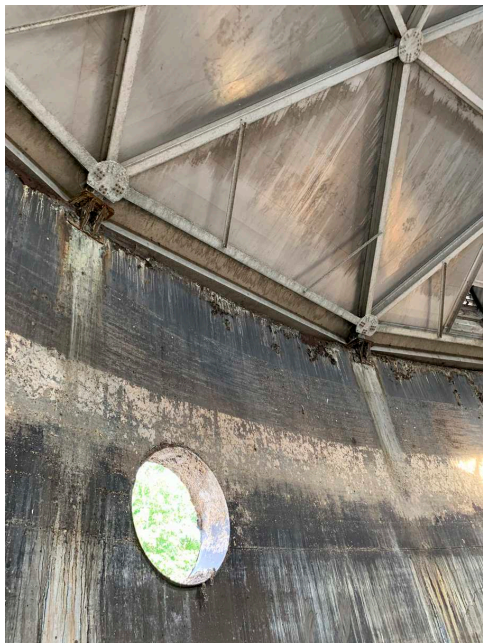
WWTP Rehabilitation East Surge Tank Corrosion Issues December 17, 2019 at 10:49:33 AM
