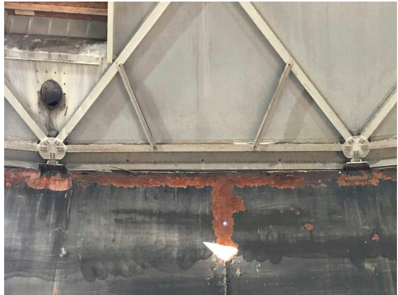
WWTP Rehabilitation West Surge Tank Corrosion Issues September 19, 2019 at 9:02:57 AM
