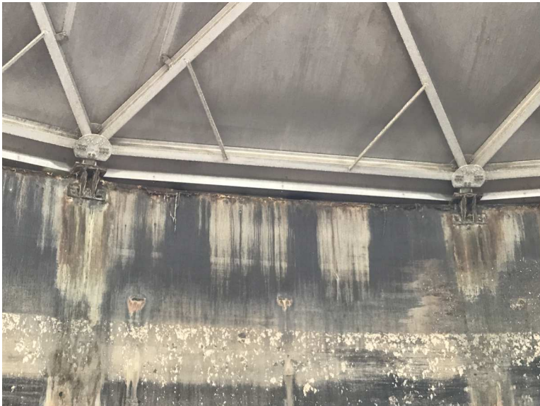
WWTP Rehabilitation East Surge Tank Corrosion Issues December 18, 2019 at 11:50:19 AM
