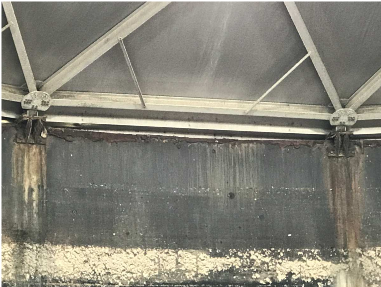
WWTP Rehabilitation East Surge Tank Corrosion Issues December 18, 2019 at 11:50:30 AM
