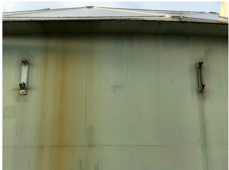
WWTP Rehabilitation West Surge Tank Corrosion Issues October 7, 2019 at 8:06:51 AM
