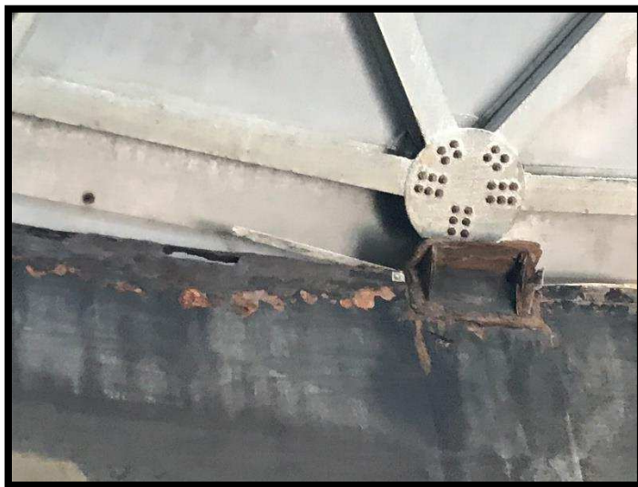
Figure 3: Dome Beam Seat Connection
