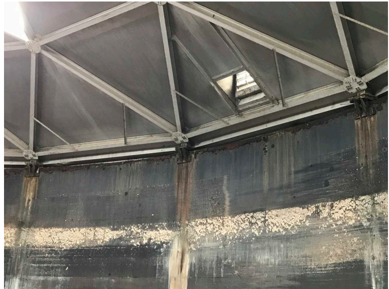
WWTP Rehabilitation East Surge Tank Corrosion Issues December 18, 2019 at 11:49:09 AM
