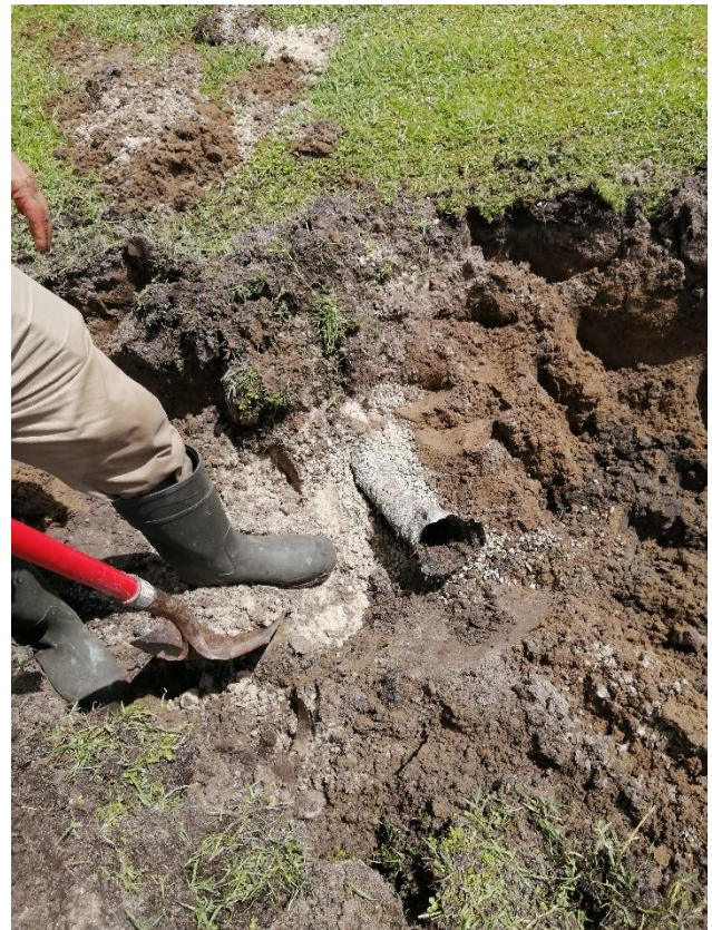
Test Pit #3: An exposed drainage pipe
