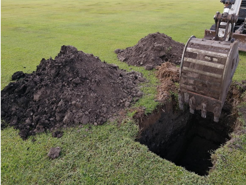
Test Pit 1: Excavated material from 0 to 6.5 ft
