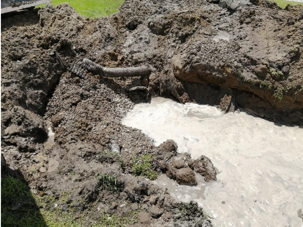
Test Pit #3: Exposed drainage and yard drain pipes, south side of the vertical drain pipe
